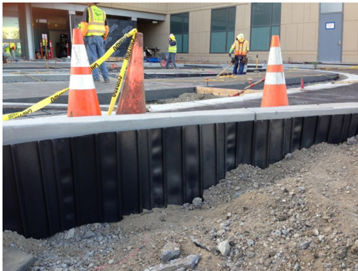
Root Solutions Installation
